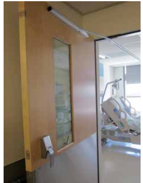
Glynn-Johnson® hospital push/pull locks and hold-opens are used on patient rooms in the new Tower hospital building.
