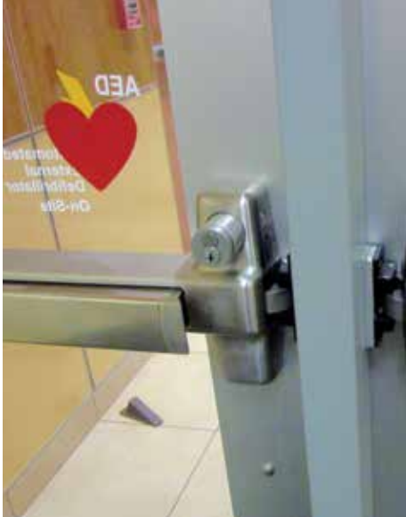
The 99 Series exit devices are preferred by Tarrant because they have a four-bolt mounting that provides a higher level of strength and security.
